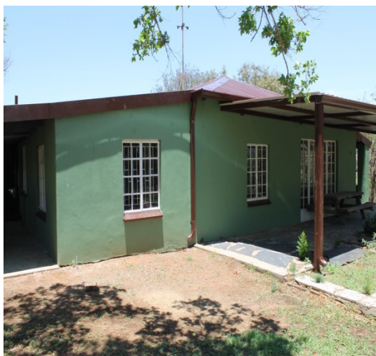
General Renovations of Schoongesight house
