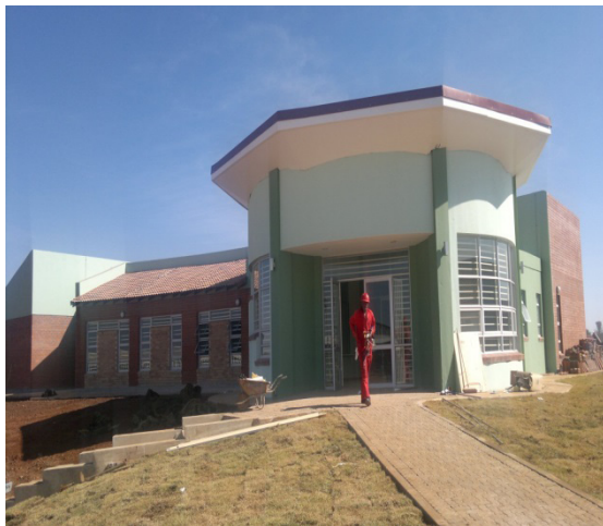
Protea Glen Aged Care, Admin Facility
