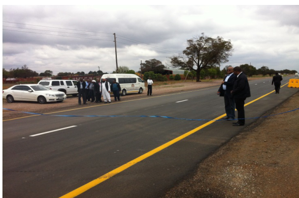
Rehabilitation of road p122/1 alternative road to e 'tolls rehabilitation of road d2129 in the Tshwane Region
