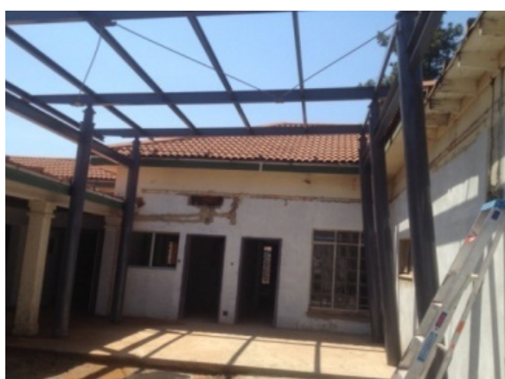
Tshwane District Hospital – TB ward: Steelworks in progress
