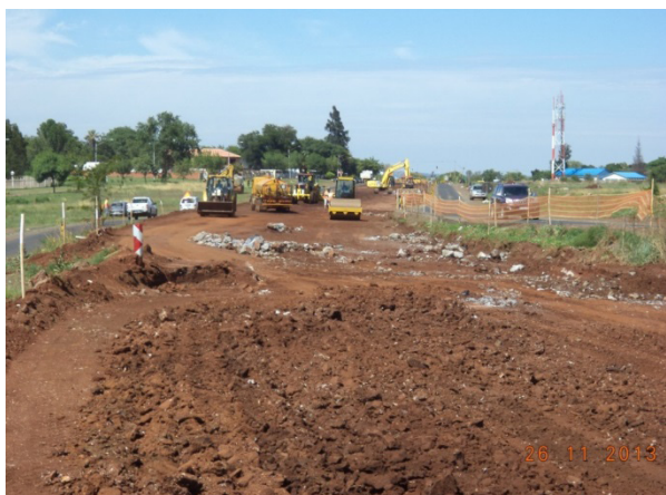
P39/1 (Laudium to Diepsloot) - During Construction
