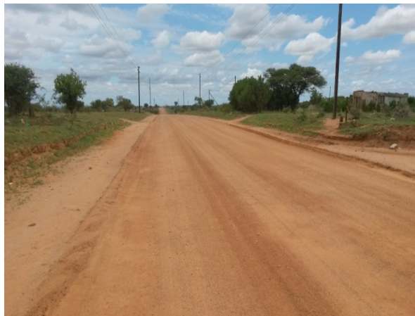
Rural Roads D620/621 Winterveldt upgrading from gravel to surface using ultra -thin concrete technology (before and after construction)
