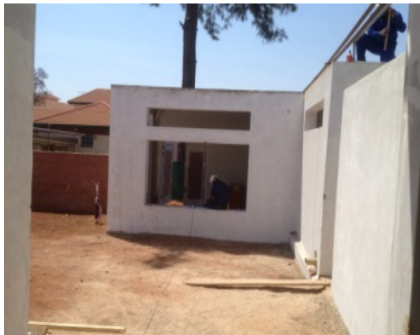
Tshwane District Hospital–TB ward: Plastering and basecoat
